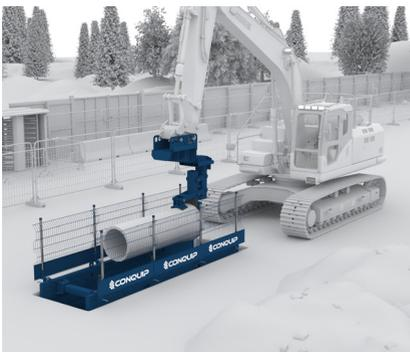
10. Lower the pipe into the Drag Box with the aid of a banksman ensuring all personnel are clear of the operation.
