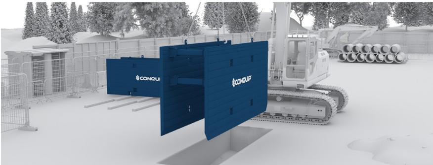
2. Using an excavator or other suitable lifting apparatus, lower the Drag Box into the trench, with a suitably rated 4 leg chain.
