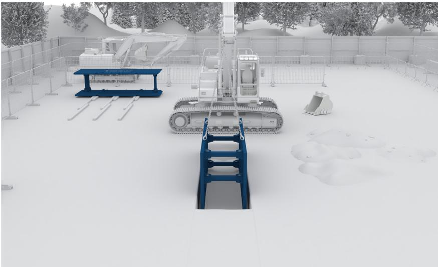
13. Return to the excavation and back fill between the panels of the base box.
