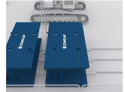
15. Carefully lift the base box out of the excavation and place on timber bearers.
