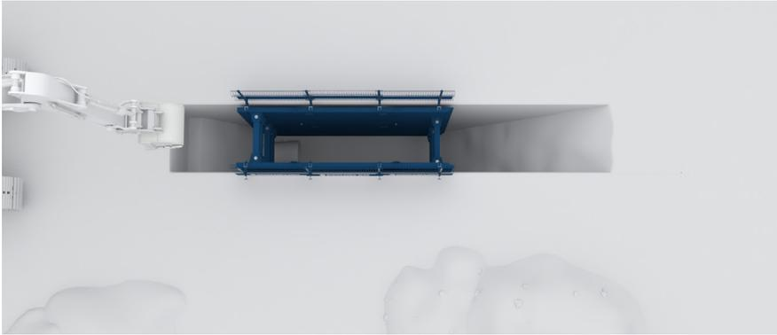
13. Backfill onto the pipes at the rear of the Drag Box.
